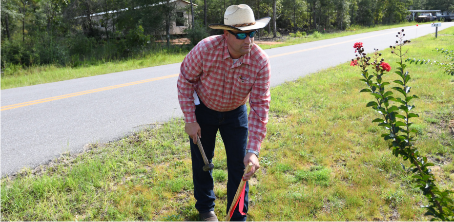
Rigby places a stake in the ground to mark the location of a future guy wire.
